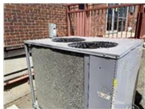
Unit GSARTU#3 is a Carrier unit Model#: 38AUZA08AOA6A0A0A0 Series#: 2022C10916 3-phase 7.5 RTU and 1 year old
