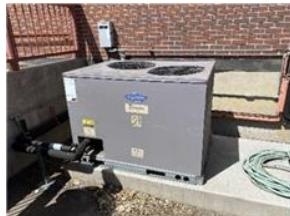
Unit GSARTU#1 is a Carrier unit Model#: 38AUZA07A0A6A0A0A0A0, Series#: 2612C90072 3-phase 6.6 RTU and 15 years old
